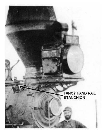
This type of handrail was also secured at the cab end by stub stanchions that were attached to the sides of the steam dome base. There were no boiler-mounted stanchions used.
